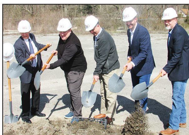
(SOUTHSIDER VOICE PHOTOS BY AL STILLEY) Groundbreaking Friday for The Jacob featured, from left, Southport Mayor Jim Cooney, Rebar Development CEO Shelby Bowen, Southport Redevelopment Commission president and former mayor Russell McClure, and Tyler Ridge II and Tyler Ridge Sr. of The Ridge Group.
