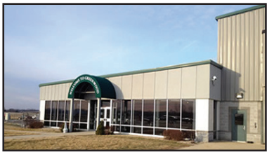
Indy South Greenwood Airport operations building is a comfortable place for pilots and visitors who come to the airport.
